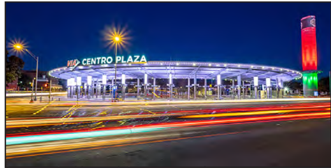
Centro Plaza Transit Center, VIA Metro Transit
