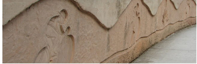
Concrete scene wall
