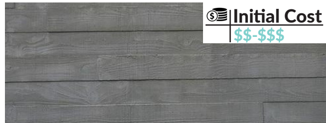
Board form concrete
