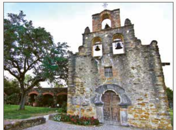
Mission Espada is one of the five Spanish Colonial missions built along the San Antonio River.
