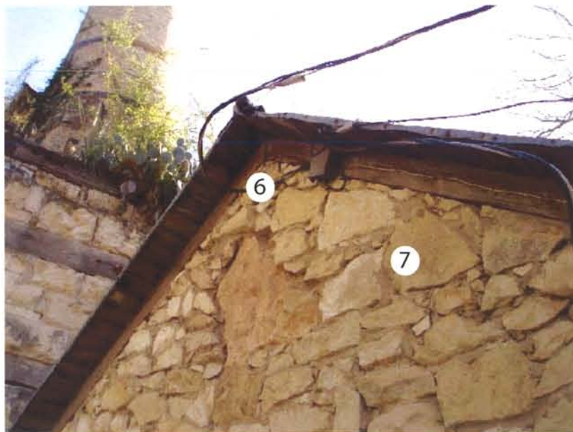
D3- Roofline at North facade
