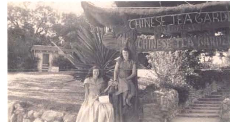
Historic image of Chinese Tea Garden Gate. The stairs appear to be constructed of stacked limestone with a layer of concrete. It is difficult to tell for certain because of the image resolution.
