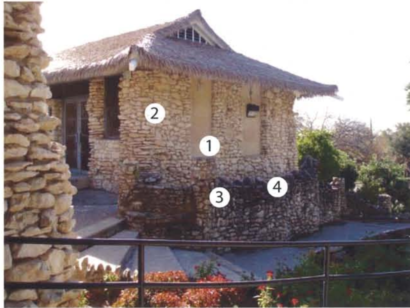
A11- Northeast corner from Pavillion
