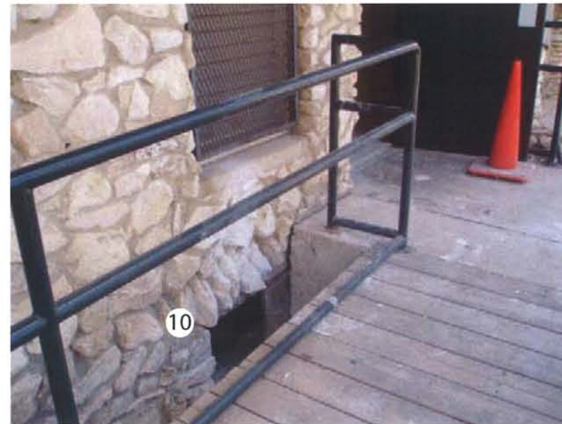
A4- East facade at accessible ramp to restrooms
