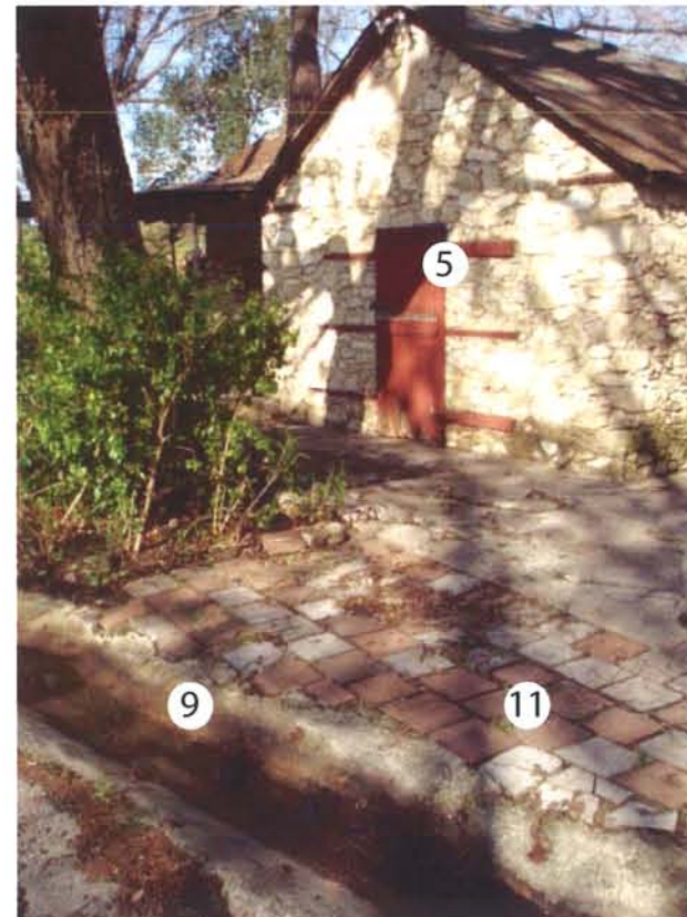
C4- Southeast corner
