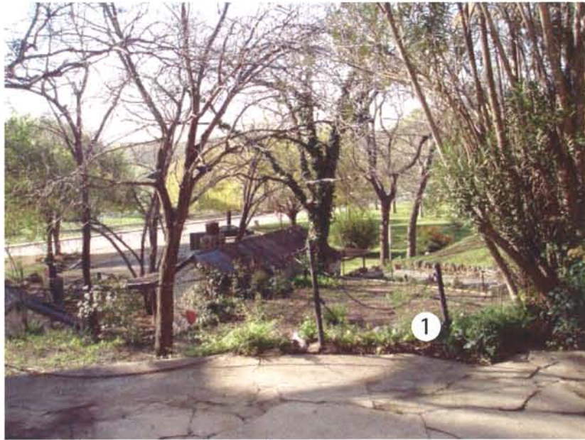
A5- Walkway at Southern edge
