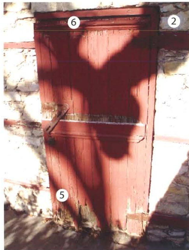
C10- Entry at South facade
