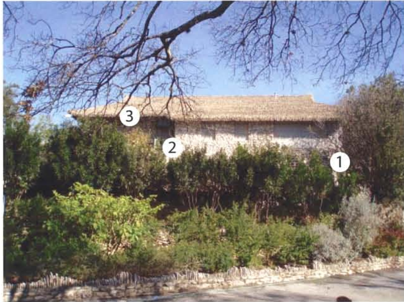
A15- West facade from road
