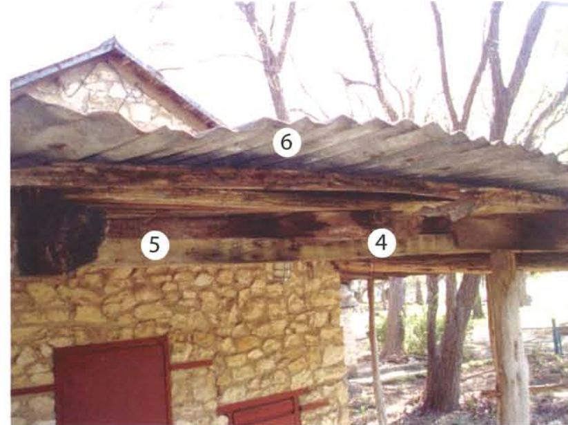
B6- Roof at West facade
