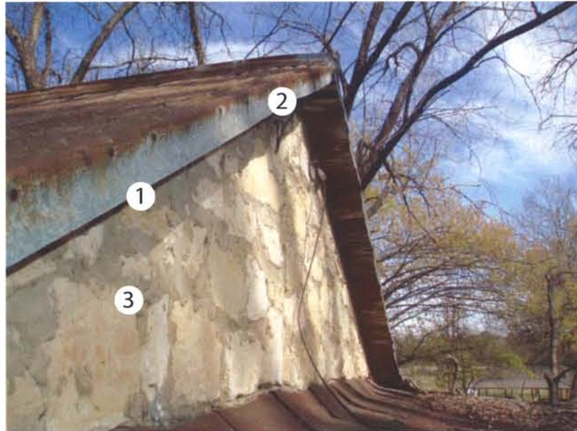
B5- Roof at West facade
