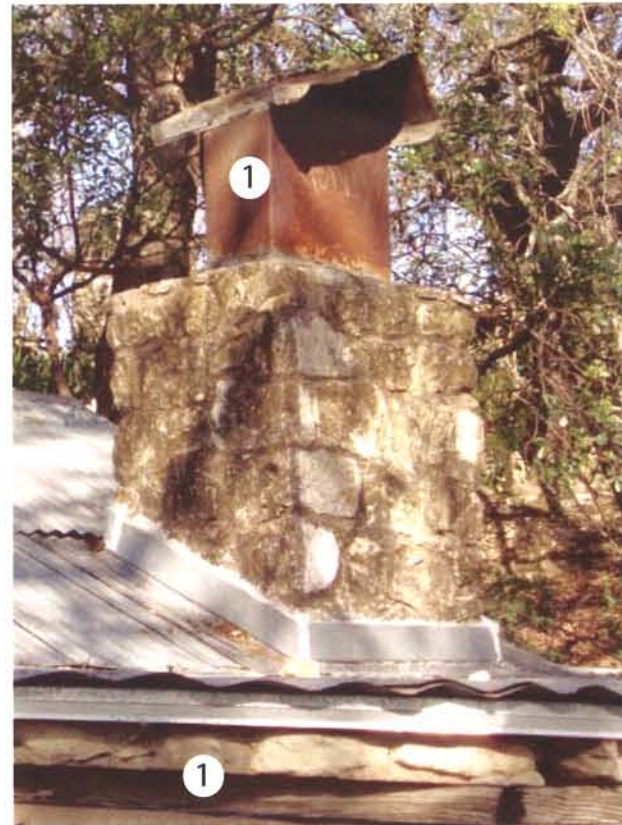
E8- Chimney at North facade
