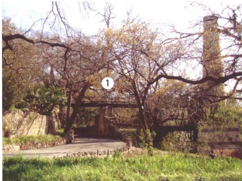
F4- Bridge from road
