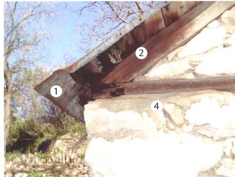
D6- Roof at Southeast corner
