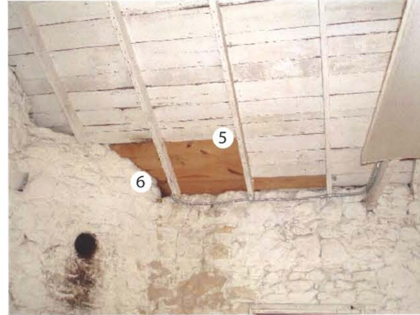
E6- Interior view of roof
