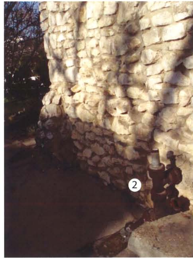
A6- South facade at rear entrance
