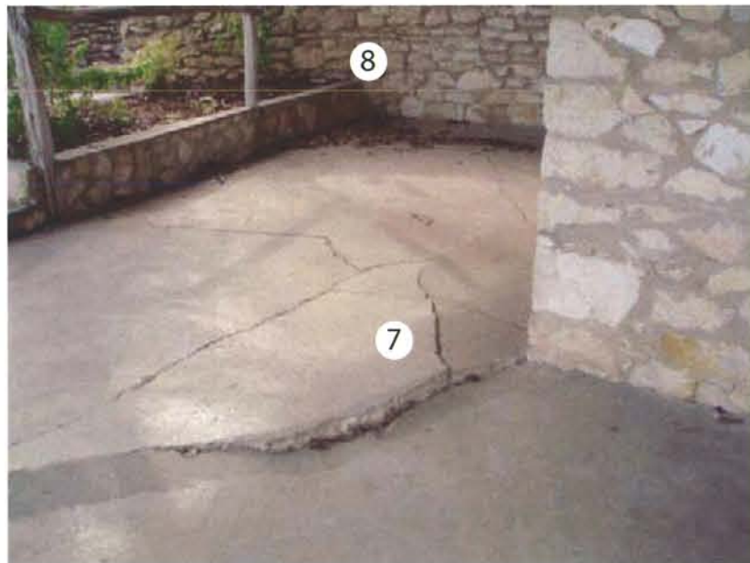
B3- Porch floor at Southwest corner
