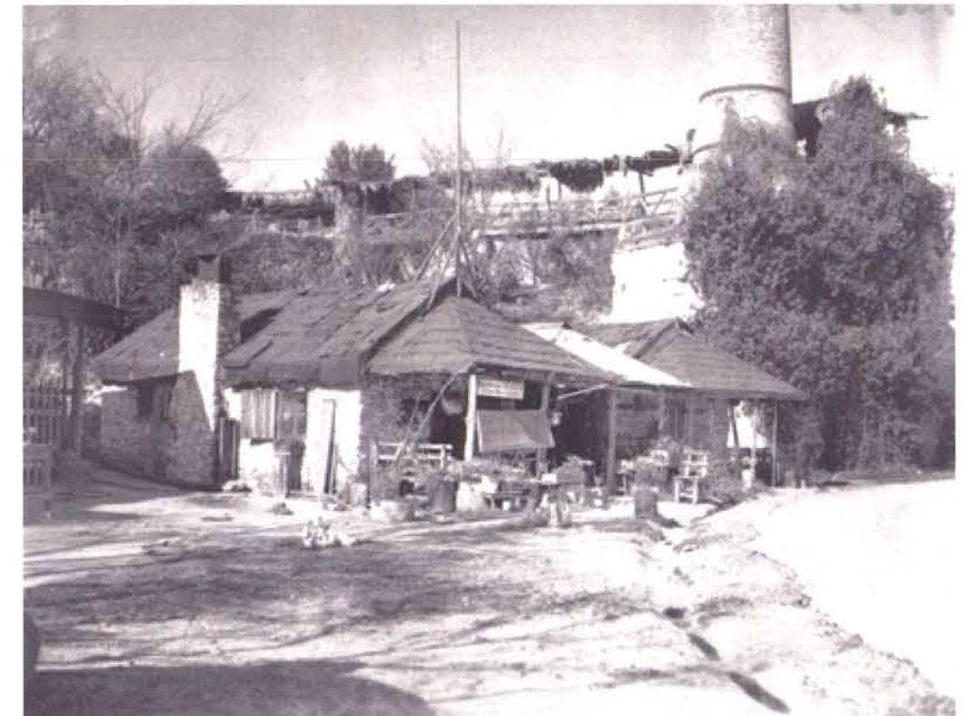
Historic image 12 shows the Mexican Village Casitas. Most of the paving was decompose granite gravel or limestone.
