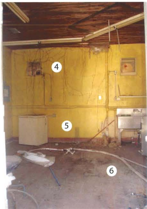
A33- Interior at second level
