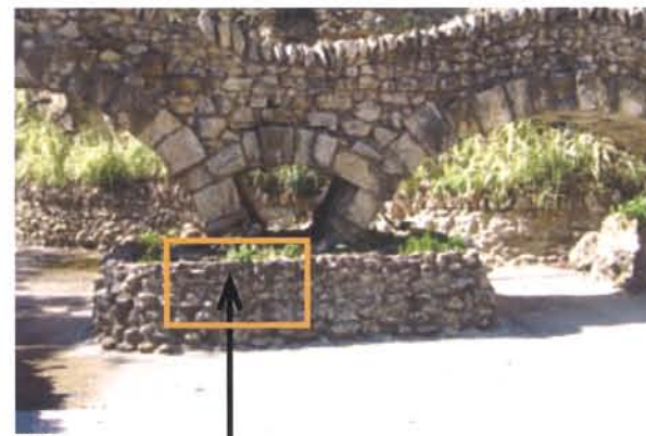
WALL CRACKED AND DETERIORATING.
