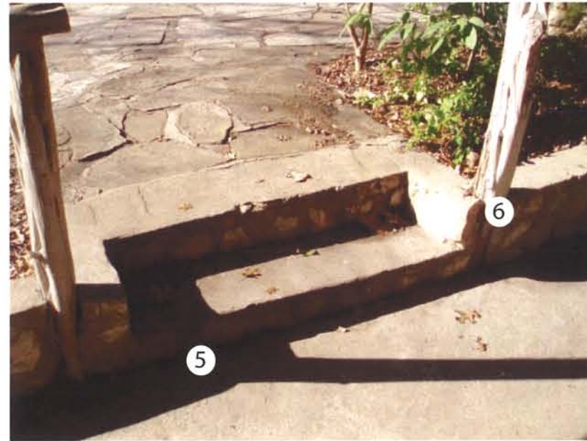
B2- Stairs onto porch at West side
