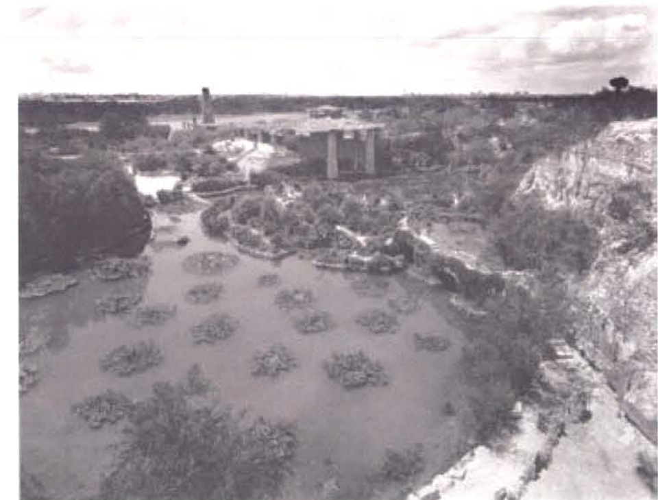
Historic image 6. Note two paths in lower right hand corner. The path was dirt, likely crushed limestone. Steps to Dragon Bridge are carved limestone. They were likely filled in with concrete over the years.
