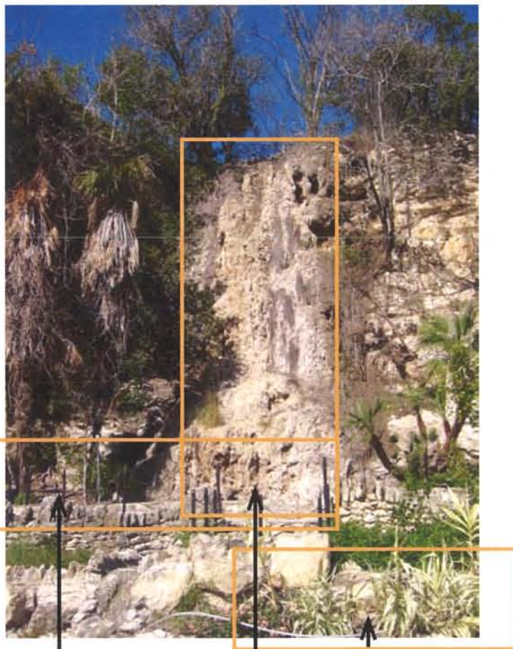
NON-HISTORIC SAFETY RAIL
