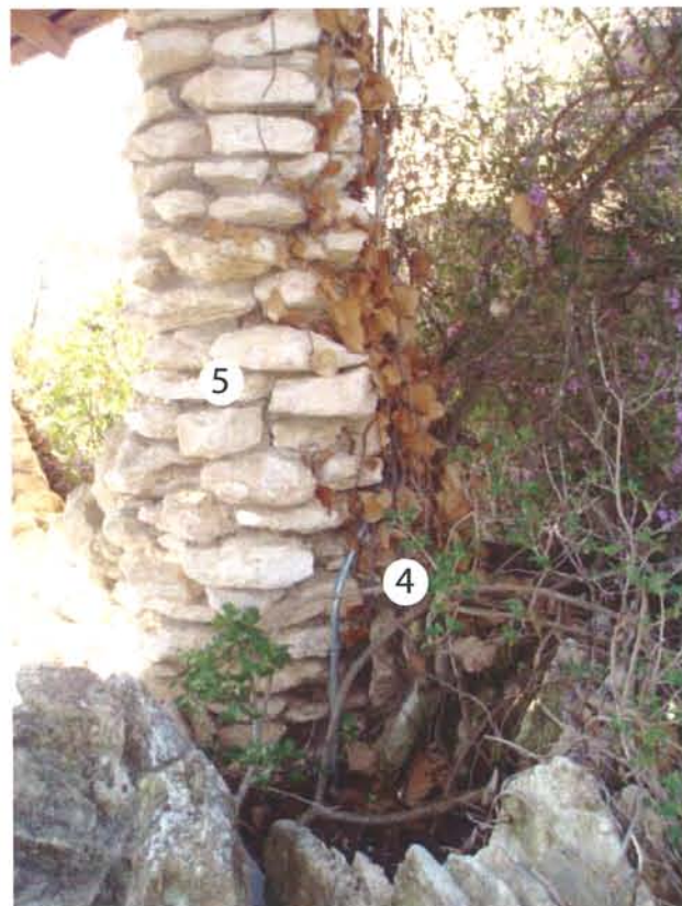
F6- Overlook column structure
