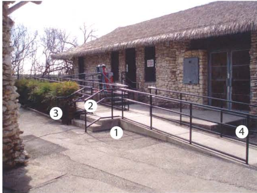
A1- East facade
