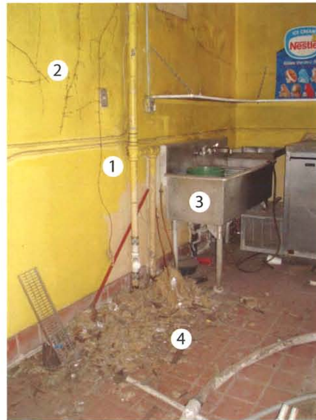
A34- Interior at second level
