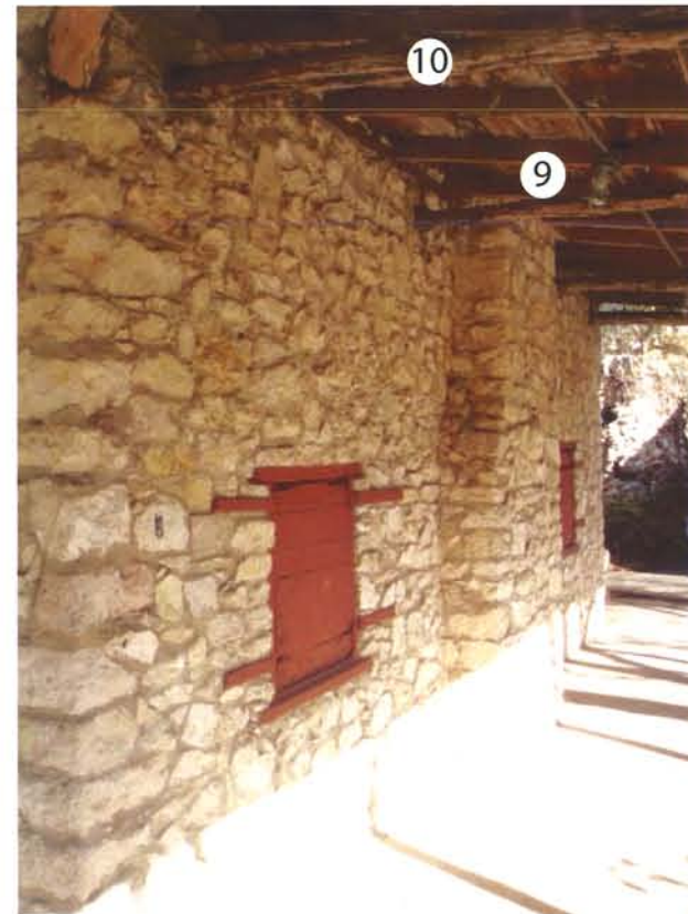
B4- South facade
