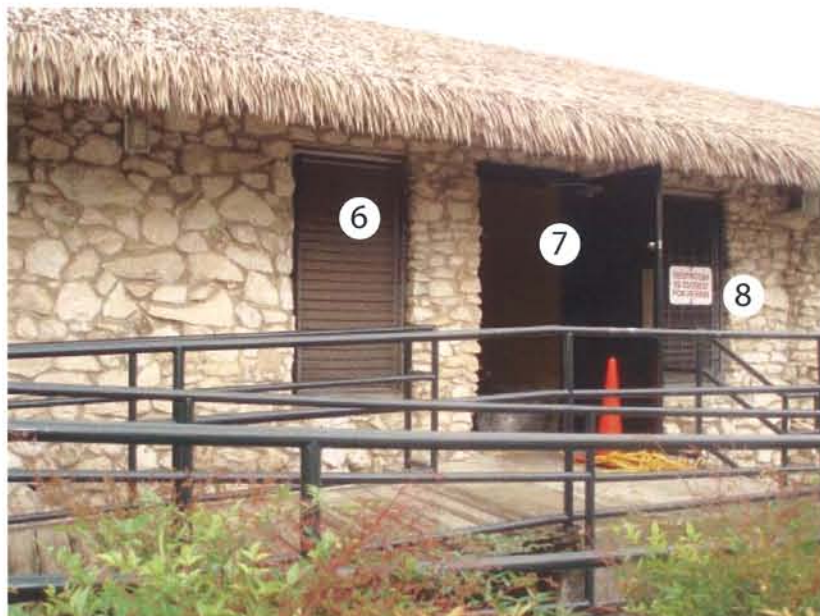
A13- East facade at restroom renovation
