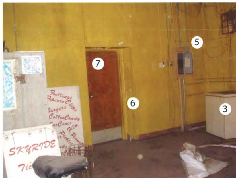
A36- Interior at second level
