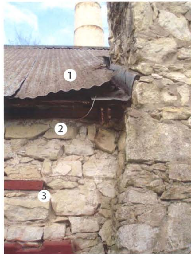
C5- West facade at chimney
