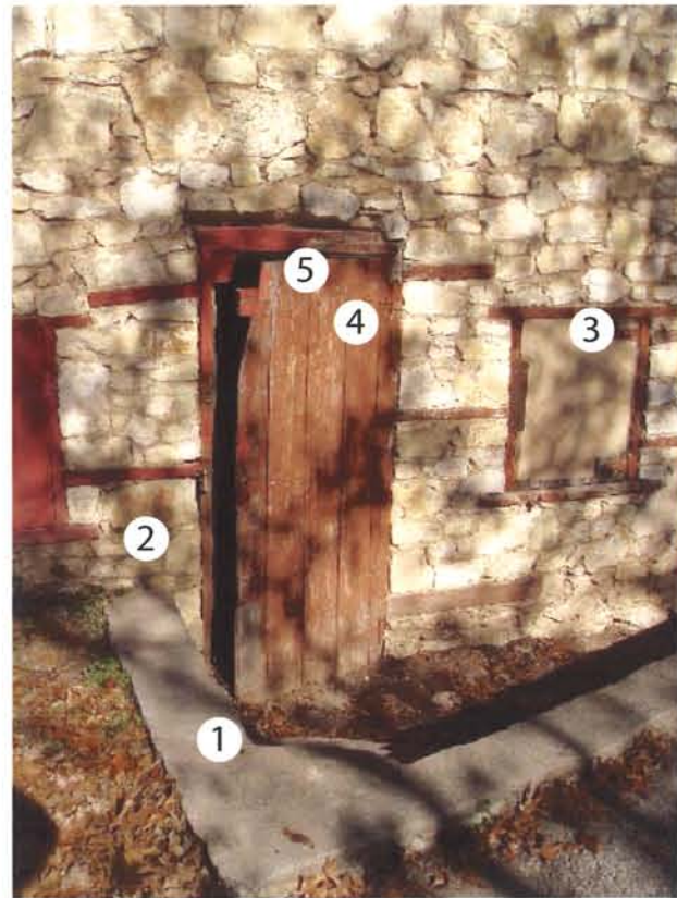
E1- Front entry at South facade
