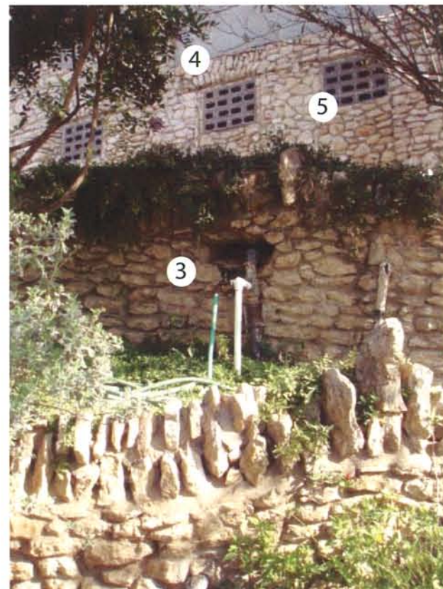
A7- Retaining wall at Southwest edge
