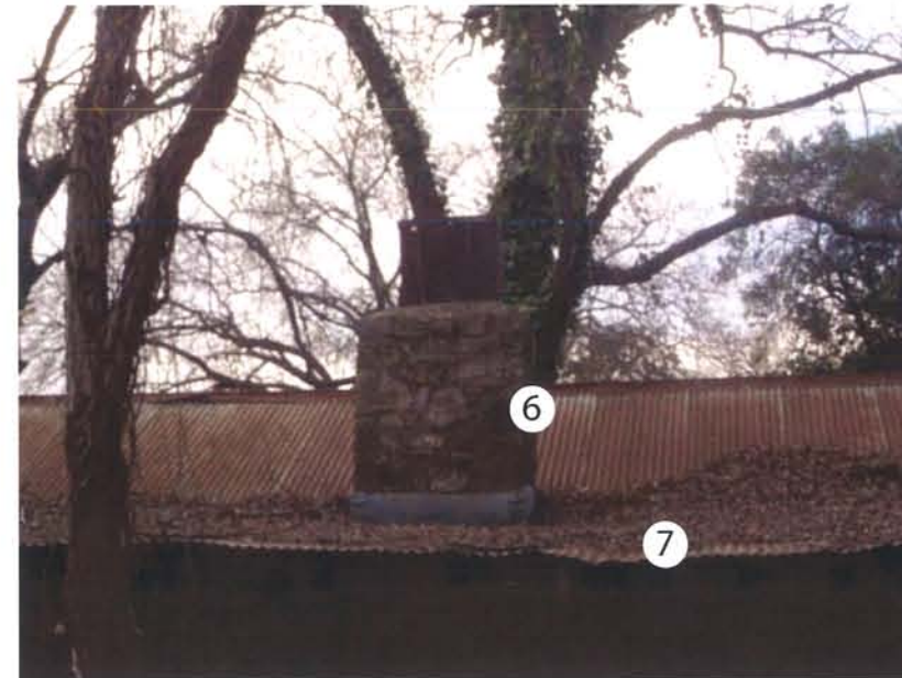
B12- Chimney at South facade
