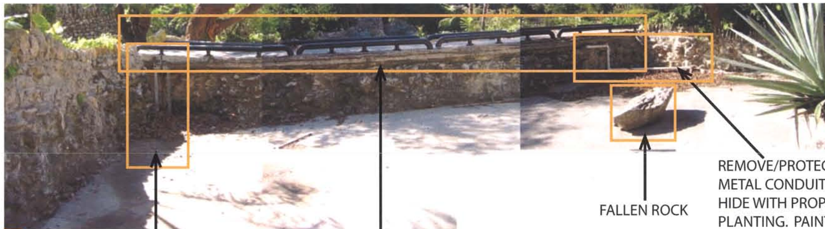
31 REMOVE PIPE. NON-HISTORIC RAILING. FALLEN ROCK. REMOVE/PROTECT METAL CONDUIT/PIPE. HIDE WITH PROPOSED PLANTING. PAINT BLACK.
