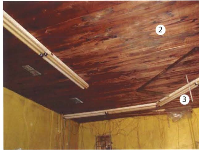
A32- Interior at second level
