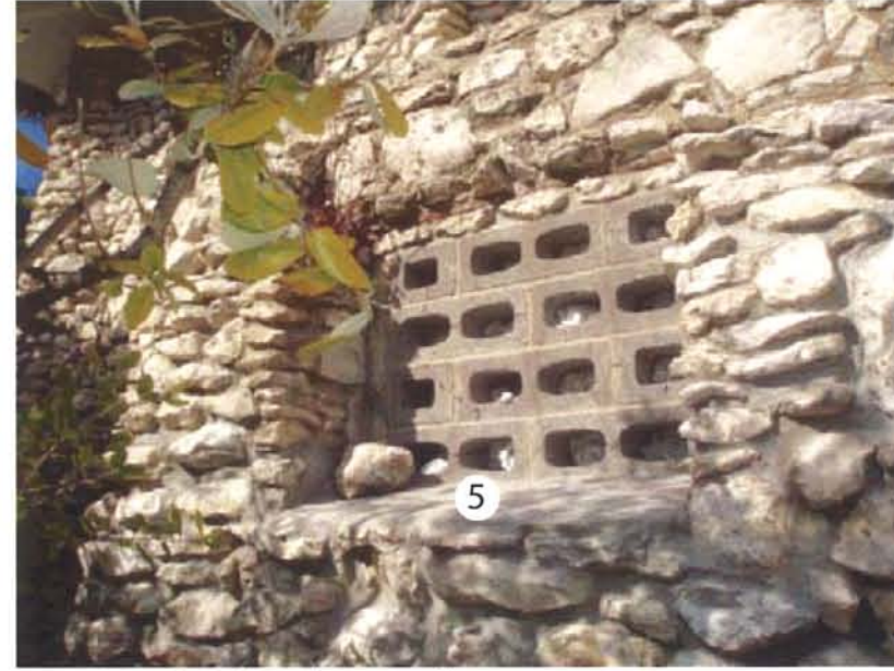
A12- West facade at lower wall
