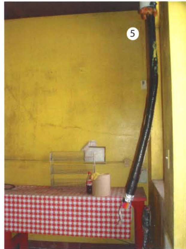
A35- Interior at second level
