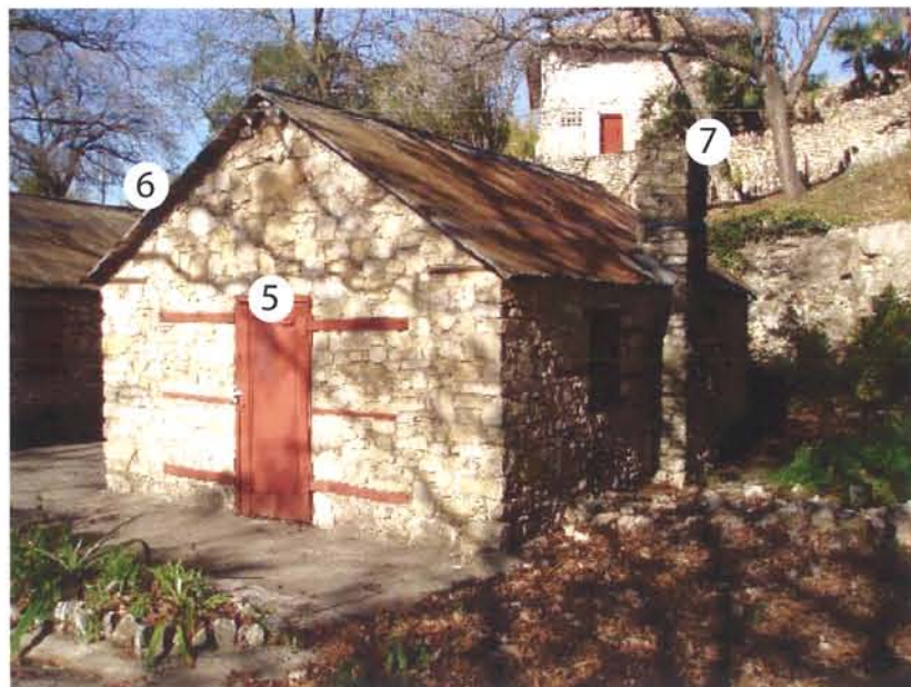
D7- South facade
