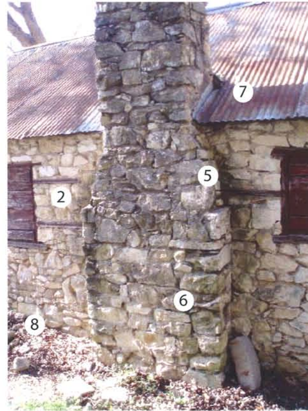
D13- Chimney at East facade
