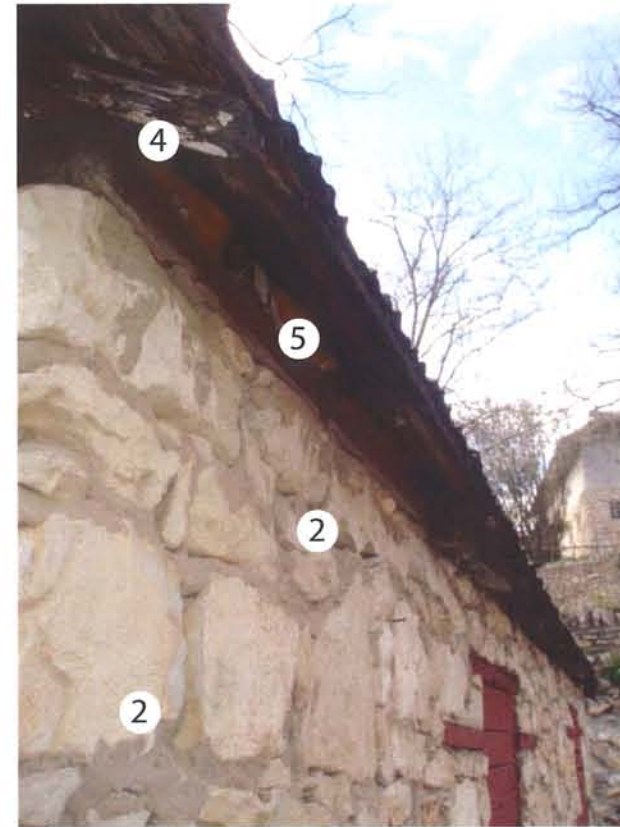
C6- Southeast corner at roof
