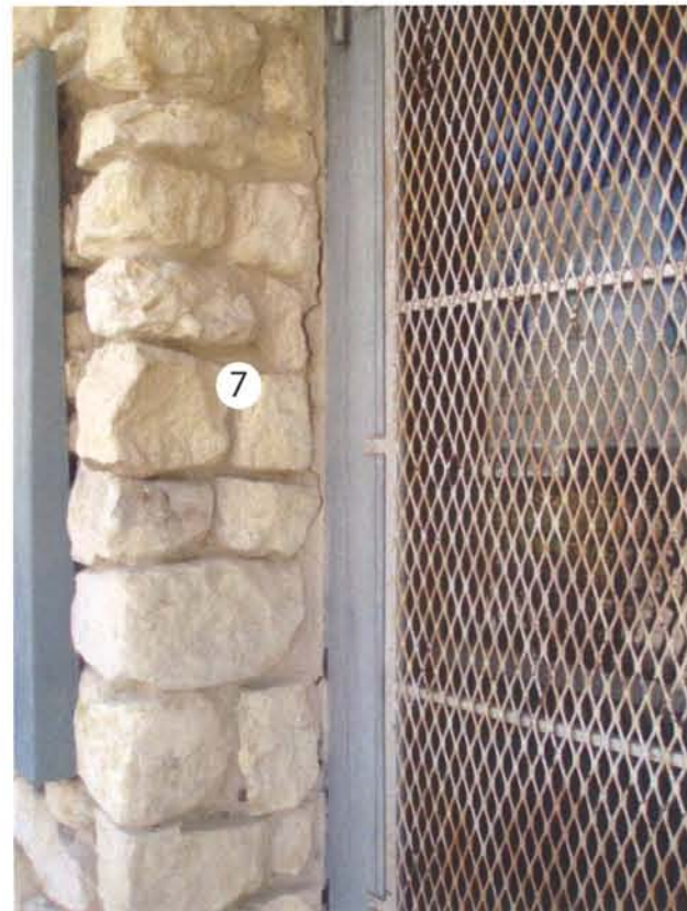
A17- East facade at concession stand
