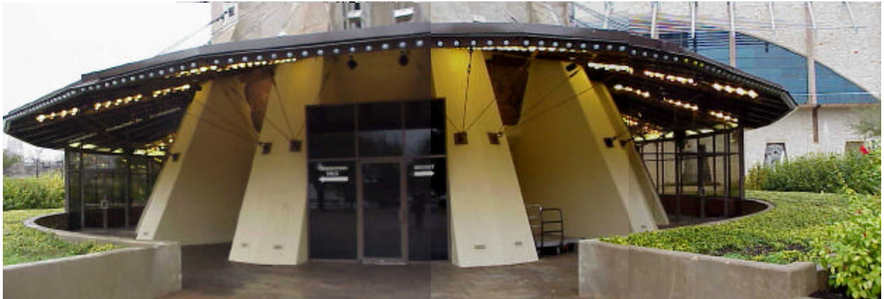
Existing Tower Base (activity level to be expanded near Tower base)
