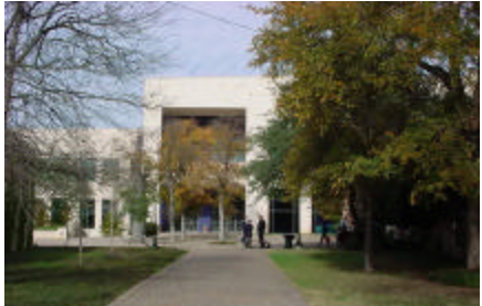
Convention Center access path
