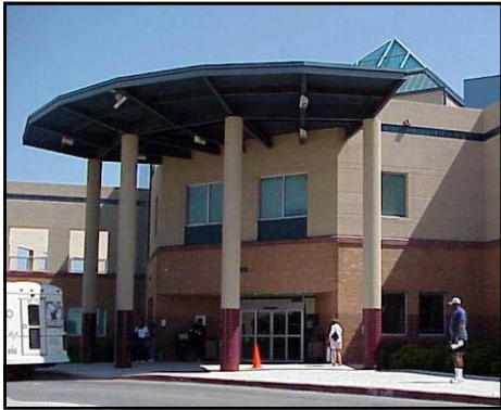
University Health clinic on Ada Street.
