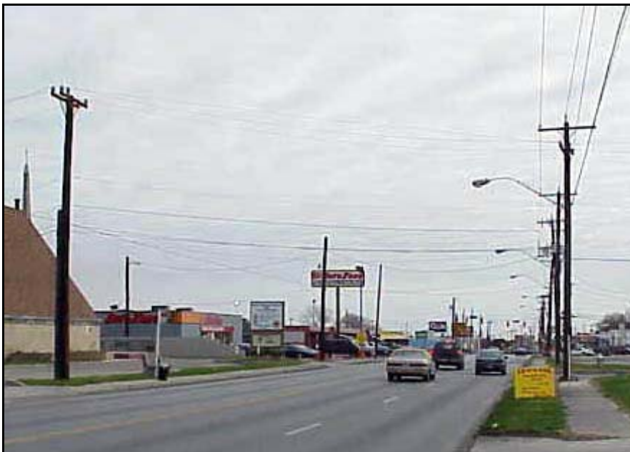
Opportunity for underground conversion of utilities along Goliad.
