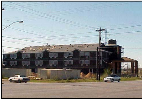
New hotel under construction at IH-37 and Military Drive
