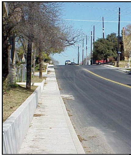
Clark Street reconstruction
