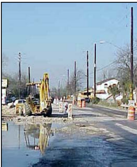
Clark Street undergoing reconstruction.
