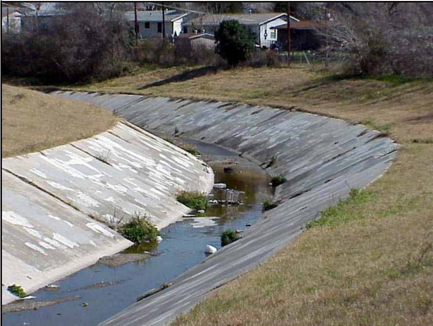
Drainage near Pecan Valley Drive and Dollarhide Avenue.
