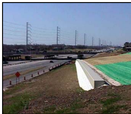
IH-37 near McCreless Mall showing new retaining wall.
