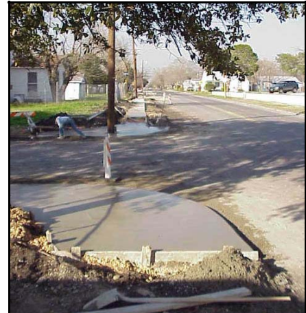
New sidewalk construction on Pine Street near Japhet Elementary School.
