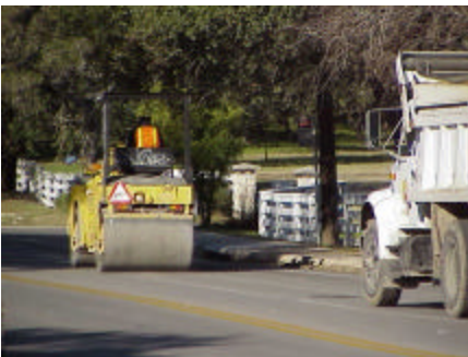
A Public Works crew working on Whitby Road
