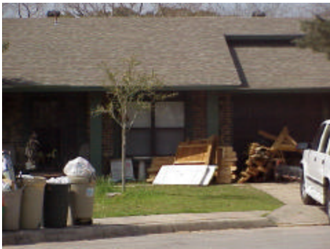
Multiple code violations at a home in Wildwood One.
