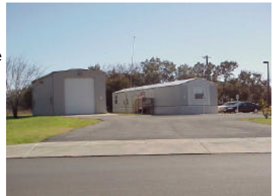
Fire Station No. 49 temporary facilities
