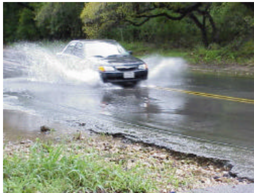
Neighborhood low water crossing
