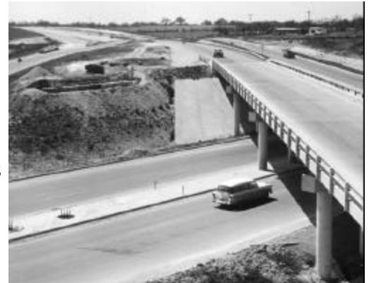
1959 image of Loop 410 construction at Bandera Road (courtesy of TxDOT)
