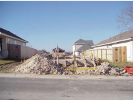
New construction at Westchase
