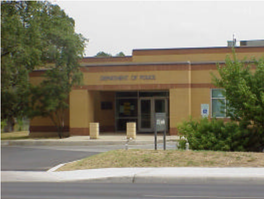
San Antonio Police Department Prue Road substation
