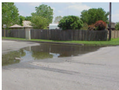
Standing water at the intersection of Rochelle and Mary Todd
