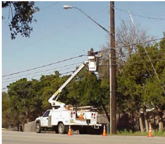
A CPS crew working on Prue Road
