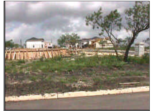
New home construction in IH 10 E corridor
