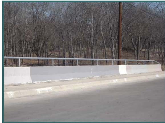
Graffiti Clean Up
