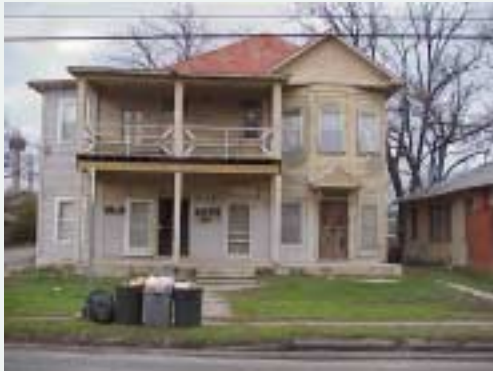
Neighborhood home in need of repair and rehabilitation.
