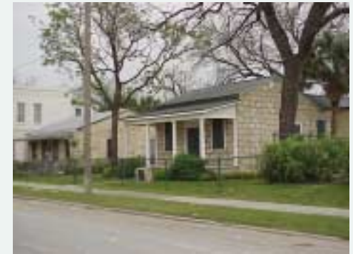
City Historic Landmark structure on Lavaca Street
