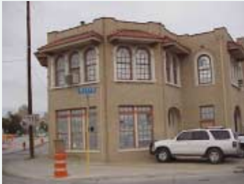
Future site of Firefighting Museum
