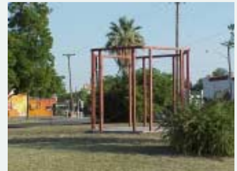
Initial construction—COSA funded Challenge Grant neighborhood gazebo
