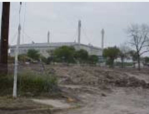
Former Victoria Courts demolitions
