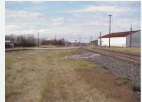
Existing conditions along Union Pacific Railroad
