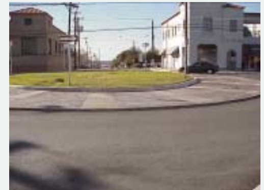
Traffic circle along McCullough Ave.
