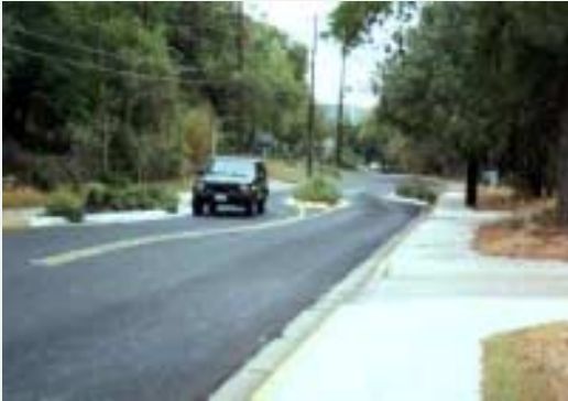
Chicane diagram (also known as deviations, serpentine, reversing curves, and twists)-one type of
