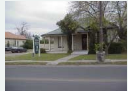
Residential structure adapted to a commercial use.
