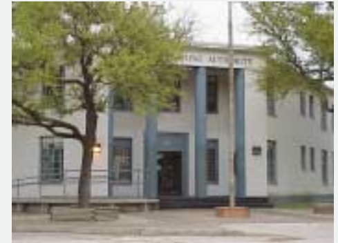
Existing San Antonio Housing Authority Building at 400 Labor St.
