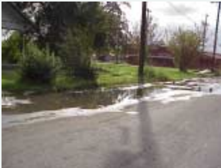
Typical drainage problems in the southern portion of the Lavaca Neighborhood
