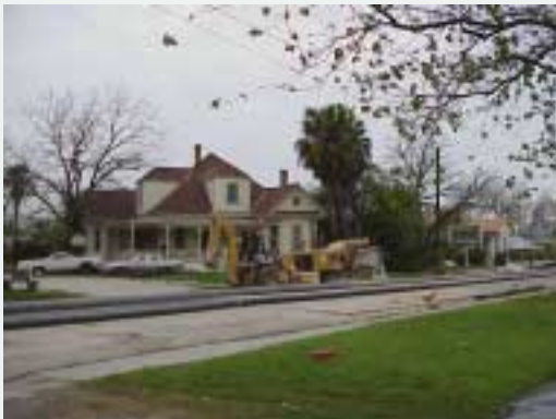
South St. Mary's Street is currently under construction.
