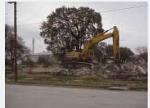
Demolition at the former Victoria Courts site
