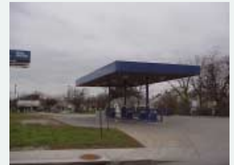
Unmanned fueling station on Florida/Carolina Sts. at IH-37
