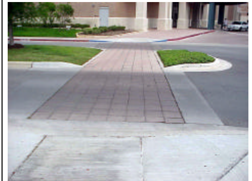
Example of a crosswalk enhancement that includes a brick paver band and a median that provides mid-street safety for pedestrians
