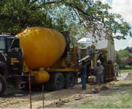
Construction crews at work in the planning area
