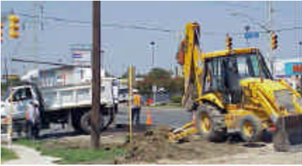
Road construction project
