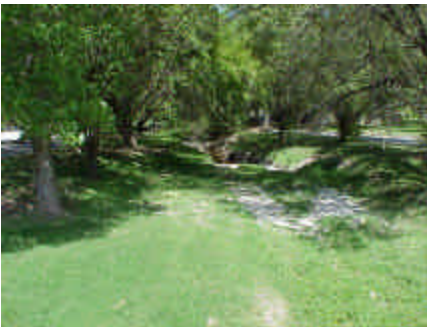
Area drainage channel
