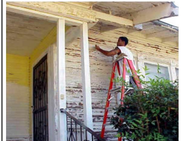
Repairing and painting a house.
