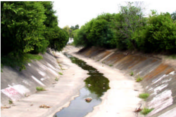
Concepcion channel at Nunes Street
