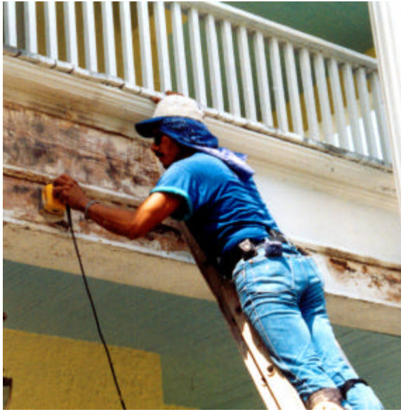
Working on a house
