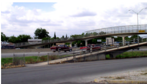
Pedestrian bridge over IH-35 from corner near the Pan American Library
