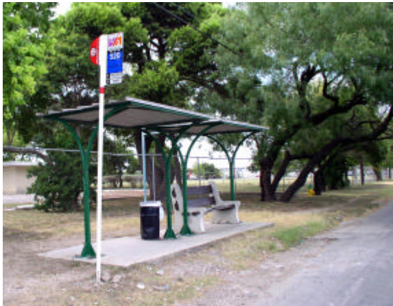
Bus shelter—Zarzamora St. at Centennial Blvd.
