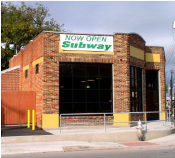
Renovated building on Nogalitos
