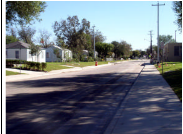
New sidewalks and paving on Hoover Street
