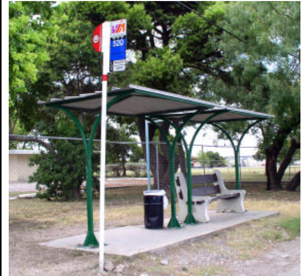
Bus stop with shelter on Zarzamora Street
