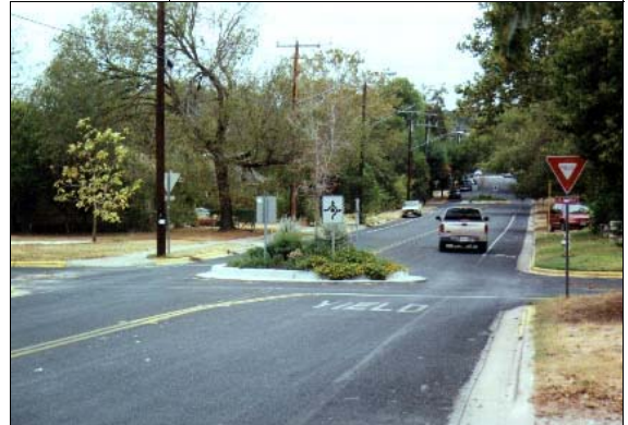
Traffic circle. Austin, Texas
