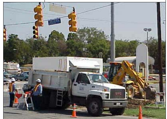
Work being done at Austin Highway and Exeter.
