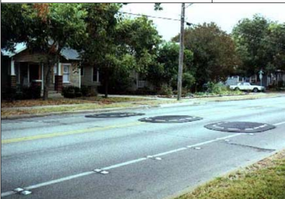
Turtles are positioned to fit the wheel base on fire trucks. Austin, Texas
