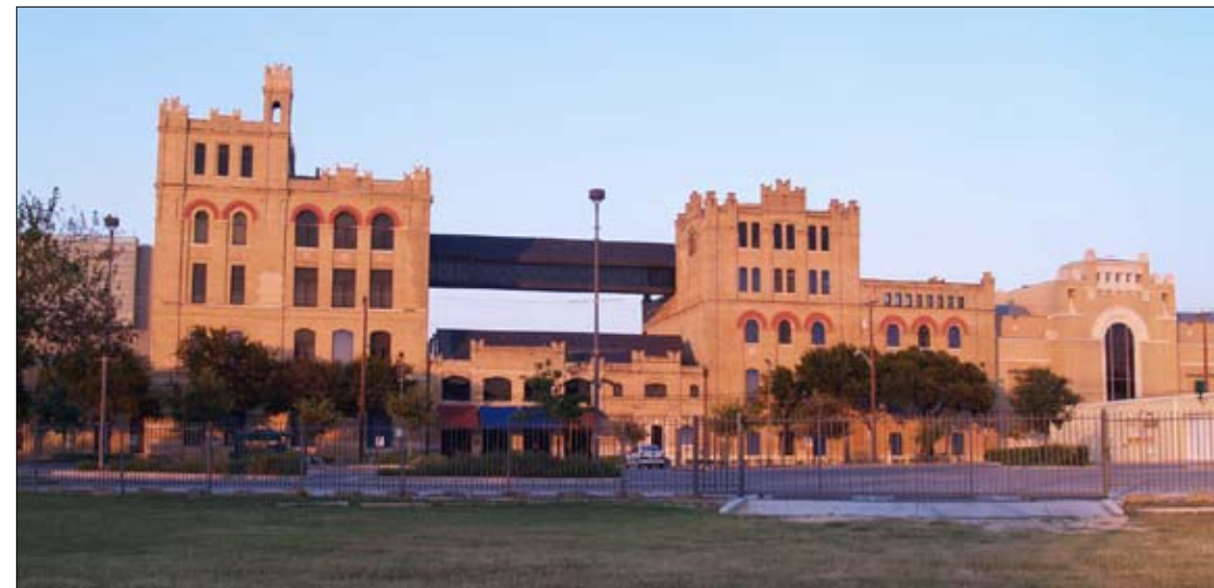
Photo of existing conditions surrounding the San Antonio Museum of Art
