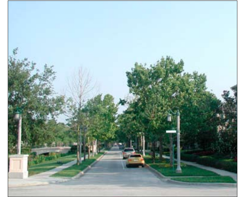
9. Streets are suitable for pedestrians: The streets are relatively narrow and shaded by rows of trees. This slow traffic and creates an environment suitable for pedestrians and bicycles. Streets are an important component of the public realm.
