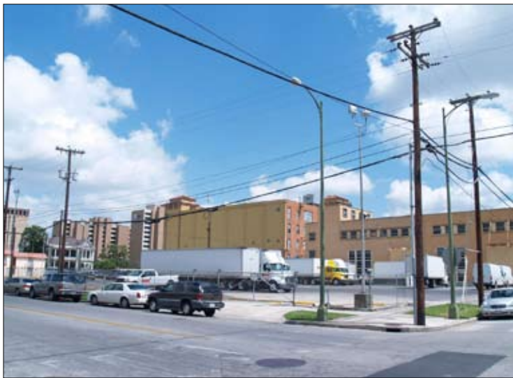
Below: An underutilized surface parking lot along Fourth
