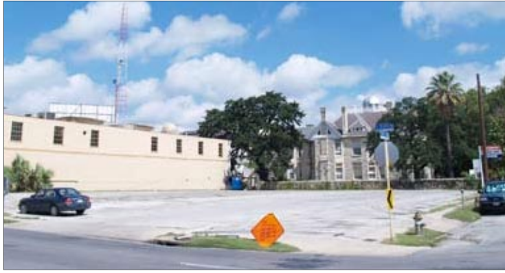
Left: Currently, the view of the Municipal Auditorium is blocked by the Radius Cafe Building
