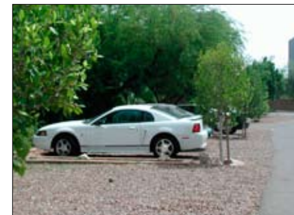
Below: Building areas of parking lots out of porous material allows direct natural drainage.
