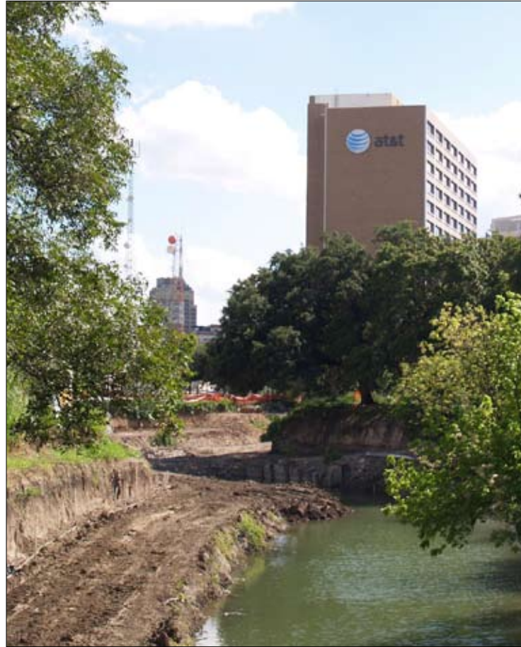
Above: San Antonio River Improvements in progress: looking south to Downtown
