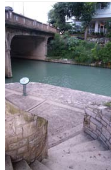
A public stairway connecting the river to the street grid
