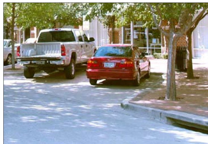
V-gutters allow storm water to flow between the parking and the street.
