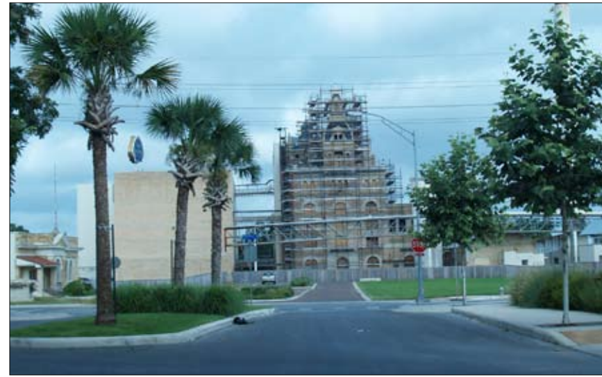
Right: Pearl Brewery redevelopment underway
