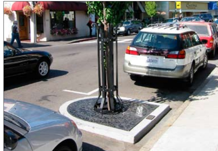
An open gutter between a curb extension and the sidewalk
