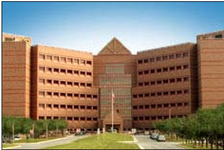
Proposed consolidated tower improvements at BAMC; Courtesy Brooke Army Medical Center
