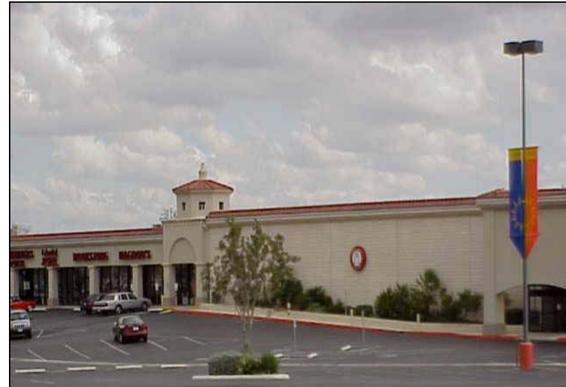
Alamo Hills Plaza on Austin Highway
