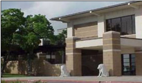
Left: Churchill High School on Blanco Rd. recently had $24.16 million in renovations and additions. Courtesy of NEISD
