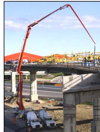
Left: Construction at Loop 410/US 281 interchange
