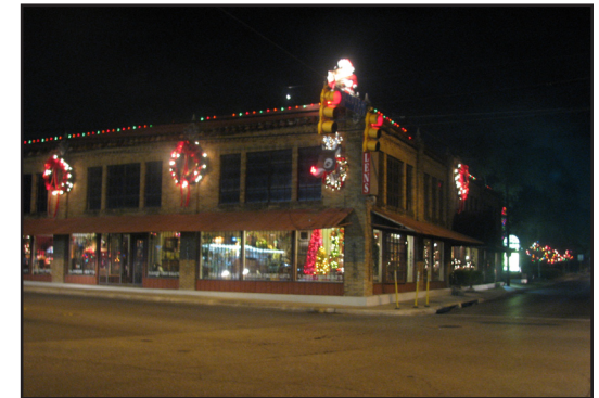
Businesses that are compatible with the neighborhood aesthetics, such as this one should be targeted for investment in the Tobin Hill area.
