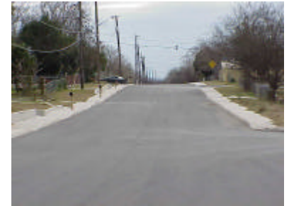
Dempsey Drive was recently reconstructed.
