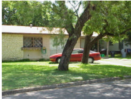
Front yard parking is a common code violation.
