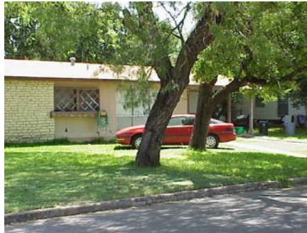
Front yard parking is a common code violation.
