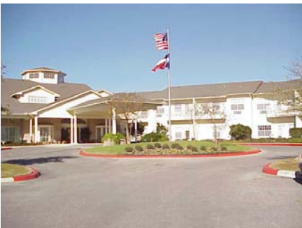
An independent living facility in Northwest San Antonio
