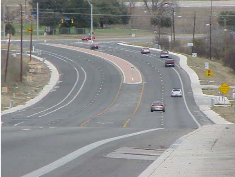
Above: Old Pearsall Road was recently reconstructed to provide additional lanes, bicycle amenities, sidewalks and bus pull-outs.
