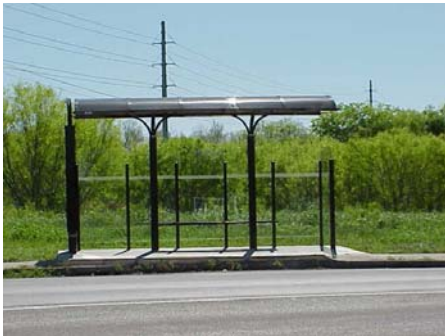
Bus shelter on Five Palms
