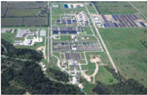
SAWS Dos Rios Water Recycling Facility
