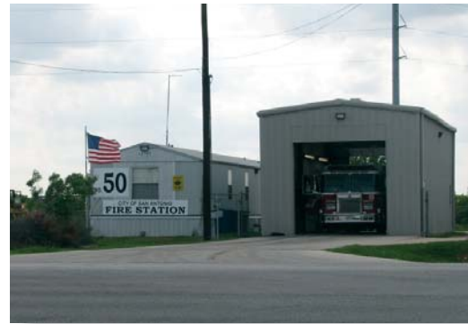
SAFD Station #50, 12703 Applewhite Rd., Note: Construction of permanent station will begin in Winter 2010.
