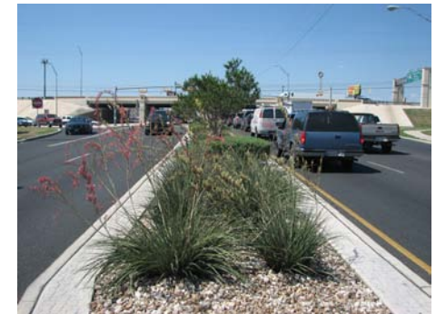
▲ Remnants of right-of-way can be transformed from an eyesore (top) to an asset (middle and bottom) with attractive, drought tolerant landscaping.
