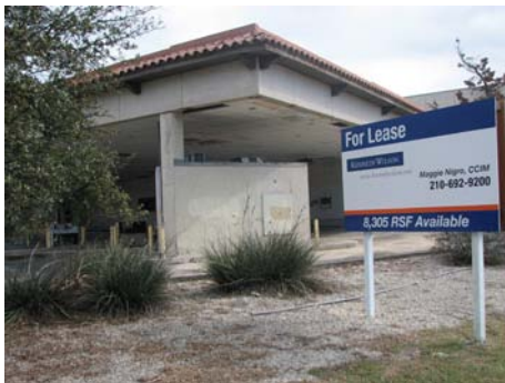
▲ Modest facade improvements at the Nacogdoches Village Shopping Center brought new regional and national tenants (before photo top, after photo middle). The rolling list of top 10 improvement opportunities includes highly visible properties such as this former Bank of America bank building (bottom).
