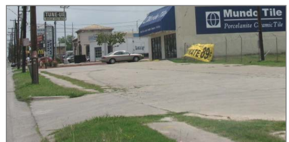
Area along Cypress in need of sidewalks and streetscape enhancements
