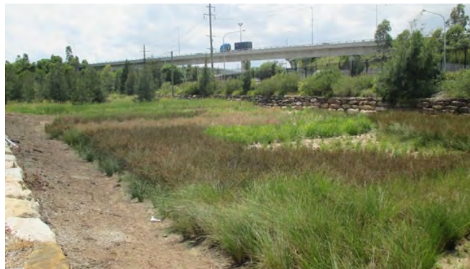
Figure A2.3b: Bioretention feature and swale in Georgia
