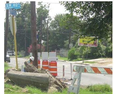
Street and sidewalk improvements along Castroville Rd.
