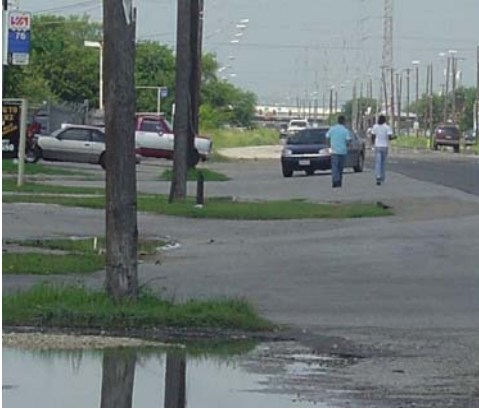
Old Hwy 90: Drainage issues after rain and lack of sidewalks
