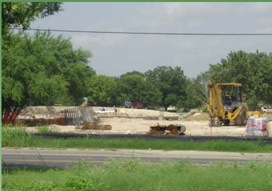
Stafford Elementary, New Construction
