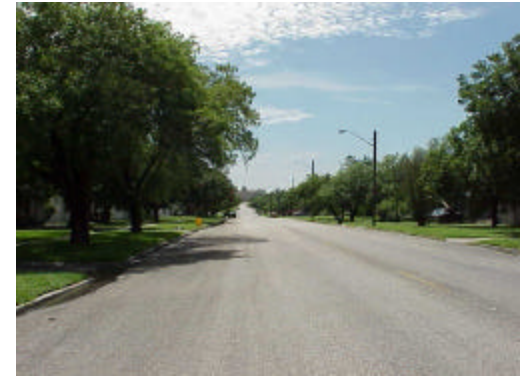
Roadway within area that consistently experiences excessive speeding.
