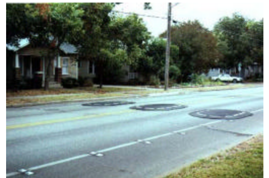
Potential traffic control measure to alleviate speeding on neighborhood streets.
