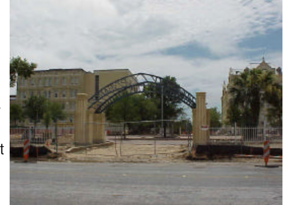
St. Mary's University Gateway Project currently under construction.
