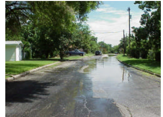
Area experiencing drainage problems in the neighborhood.
