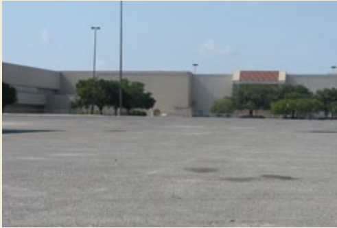
The top image shows Windsor Park Mall during a busy shopping day when the mall was a regional draw. The bottom image shows the vacant mall today. The former mall is being transformed into the corporate headquarters for Rackspace Hosting.
