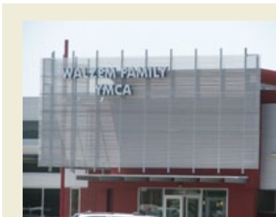
The new Walzem Family YMCA provides recreational opportunities to community members. The YMCA is the only full service recreational center in the immediate vicinity that is open to community members.
