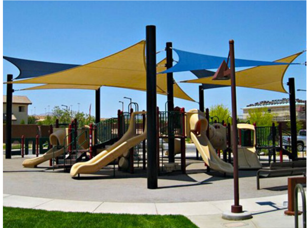
Shaded Playground Equipment
