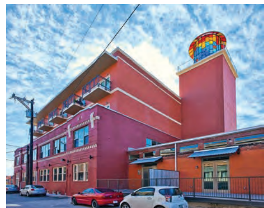
IDZ Example: Steel House Lofts
