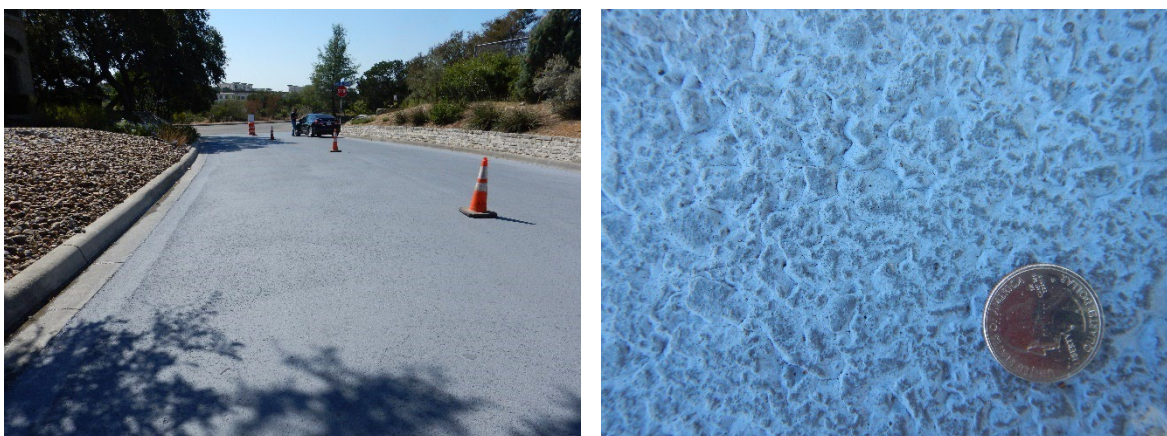
Figure 23. Photos of Frontier Hill treatment with GuardTop Iron – Light.
