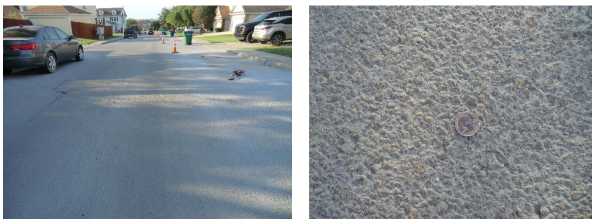
Figure 15. Photos of Rebeccas Trail treatment with Seal Master.
