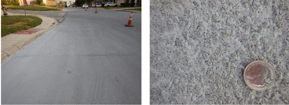
Figure 14. Photos of Mountain Star treatment with Seal Master.
