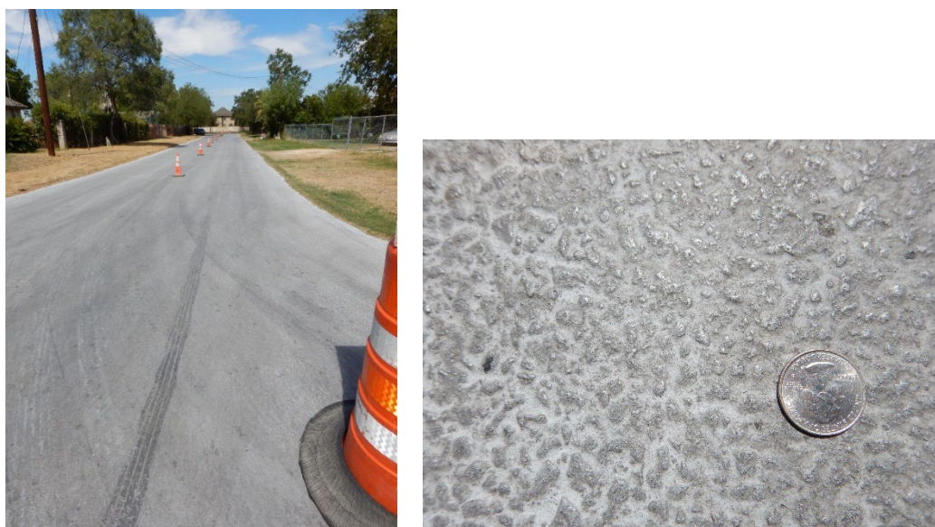
Figure 12. Photos of Lucinda St. treatment with GuardTop Iron -Dark.
