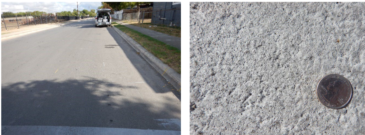
Figure 17. Photos of SW 21 st St. treatment with Seal Master.
