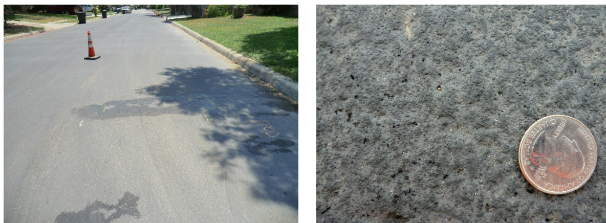
Figure 19. Photos of Spiral Creek treatment with GAF Streetbond.
