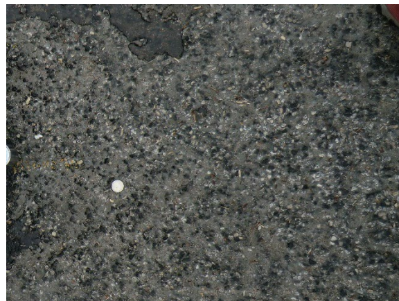
Figure 25. Photos of Encino Ridge St. treated section with Pavement Tech (top) and Encino Grove control section (bottom).
