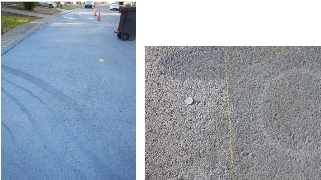
Figure 29. Photos of Villa Mercedes treatment with GuardTop Iron - Light.
